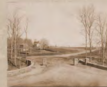
Cadwalader Park entrance, c. 1892. In the background are some of the farm buildings that were part of the Ellarslie estate.
