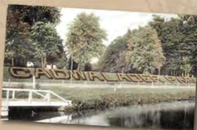
For many years, the canal embankment at Cadwalader Park featured flowerbeds. Mules would have traveled the canal towpath pulling boats.
