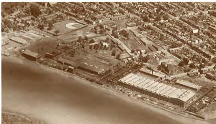
An aerial view of the American Bridge Company works in 1928. [Trenton Public Library]
