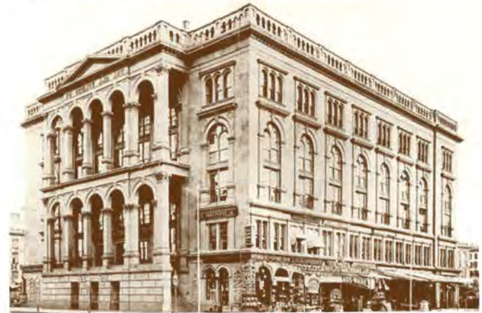
A view around 1860 of the Cooper Union building, constructed with wrought-iron I-beams made at the Trenton Rolling Mills.
