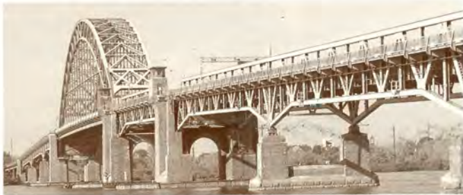
Built in 1928–29, the Tacony-Palmyra bridge over the Delaware River was one of many spans for which the American Bridge Company supplied structural steel. [Hunter Research, Inc.]
