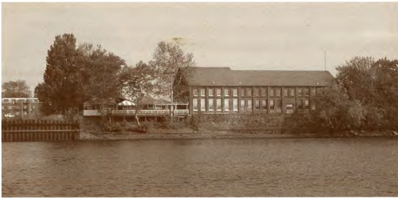
A modern view of the New Jersey Steel and Iron Company machine shop, built in the early 1870s, now adapted into a restaurant. [Hunter Research, Inc.]
