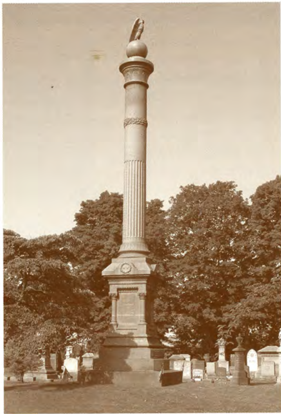
The McClellan monument positioned on the main axis and at the high point of the cemetery. [Hunter Research, Inc.]
