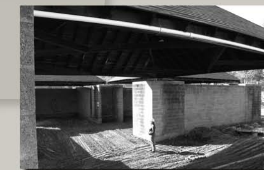
Bath House restoration, 2010.
