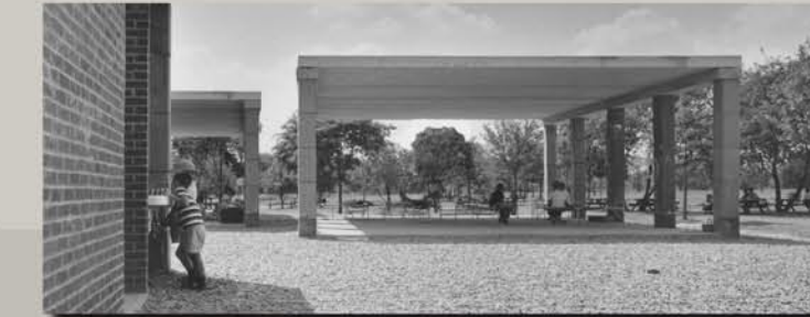
The Day Camp Pavilions were part of Kahn's JCC campus. Two of the most deteriorated of the four pavilions were fully documented, demolished and then reconstructed as part of a restoration project in 2010.
