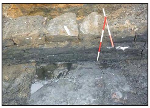
Photograph 3.12. Detailed view looking northeast showing the mortared stone masonry of the perimeter wall and floor of the late 19th/early 20th-century turntable [Structure 71] in Remedial Area 15 (PHE Area 2); scales in feet and tenths of feet (Photographer: Joshua Butchko, December 2016) [HRI Neg. #16008/D7:215].
