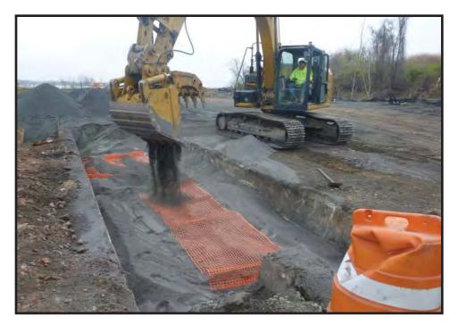
Photograph 3.47. View looking east showing the western extension of Remedial Area 15 (PHE Area 2) undergoing backfilling with gravel remedial fill; orange plastic snow fencing was placed within the fill to alert future excavators of sensitive archaeological remains below (Photographer: Joshua Butchko, April 2017) [HRI Neg. #17023/D1:707].
