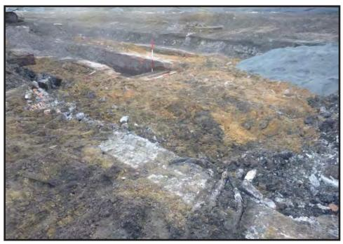
Photograph 5.21. View looking southeast showing the western end of Remedial Area 17 (PHE Area 1); the brick and stone foundation in the foreground is part of the machine shop [Structure 43]; one of the brick ash pits lies beyond within the machine shop interior; remediation in this area occurred within historic fill and contaminated natural sands to a depth of three feet (deeper within the ash pit); scales in feet (Photographer: Joshua Butchko, December 2016) [HRI Neg. #16008/D7:454].
