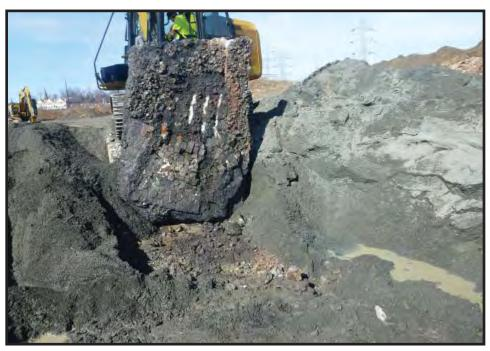
Photograph 3.28. View looking west showing remnants of the mid-19th-century turntable's brick floor [4, 6, 16] attached to the underside of the ash pit's concrete floor [2] (Photographer: Joshua Butchko, April 2017) [HRI Neg. #17023/D1:124].
