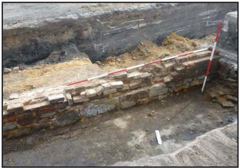
Photograph 3.44. Detailed view looking south showing the mortared stone and brick foundation [22] that supported the southern side of the approach track leading into the mid-19th-century turn-table; scales in feet and tenths of feet (Photographer: Joshua Butchko, April 2017) [HRI Neg. #17023/D1:672].
