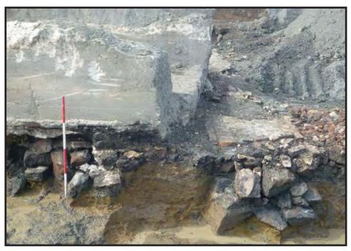
Photograph 3.36. Detailed view of part of a cross-section through the turntable pit looking northnorthwest; this view is an easterly continuation of that shown in Photograph 3.35 and shows the brick and stone foundation for the band of brickwork [16] in the turntable floor (for supporting balance wheels), with crushed stone and brick rubble fill [6] to the right; scale in feet (Photographer: Joshua Butchko, April 2017) [HRI Neg. #17023/D1:370].
