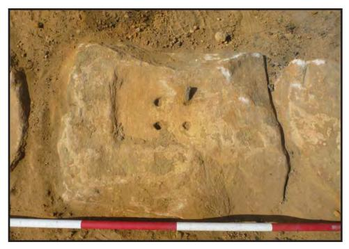
Photograph 4.8. Close-up view of typical four-hole stone sleeper, or junction block, showing oneinch diameter holes drilled to receive fastening trenails and spikes; one spike still in place; traces of the rectangular outline for the setting for the locust chair or plate are just visible surrounding the drill holes; scale in feet (Photographer: Joshua Butchko, April 2017) [HRI Neg. #17023/D1:450].
