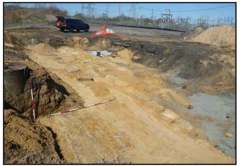
Photograph 4.10. View looking west across the western end of Remedial Area 16 (Area 3) showing the two parallel lines of packed gravel and lines of stone sleepers; the two lines of gravel, spaced approximately five feet on center, are interpreted as part of the original Camden and Amboy Railroad rail bed dating from the 1830s and would have supported standard gauge track; scales in feet and tenths of feet (Photographer: Joshua Butchko, April 2017) [HRI Neg. #17023/D1:552].
