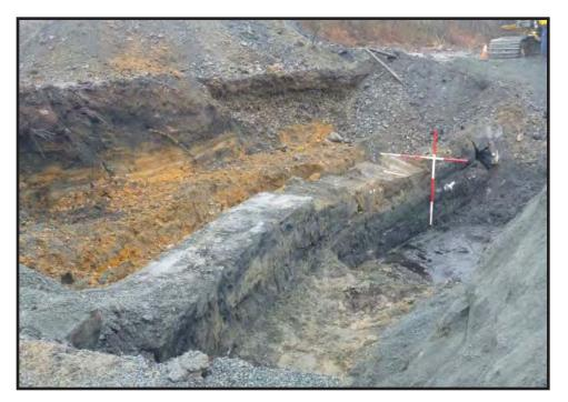
Photograph 3.11. View looking east showing a portion of the stone perimeter wall of the early late 19th/20th-century turntable [Structure 71] in Remedial Area 15 (PHE Area 2); note how this structure is set down into a construction bed of redeposited natural sands; scales in feet (Photographer: Joshua Butchko, December 2016) [HRI Neg. #16008/D7:216].
