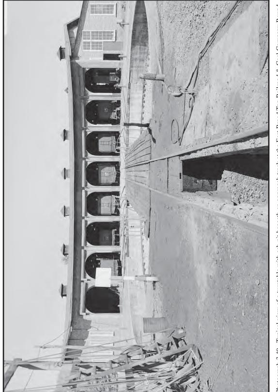
Photograph 3.49. Typical view of a turntable with ash pit beneath an approach track at the East Broad Top Railroad & Coal Company Round-house, Rockhill Furnace, Huntingdon County, Pennsylvania (Source: Boucher 1986) [HAER PA, 31-ROCFN, 1B--8]).
