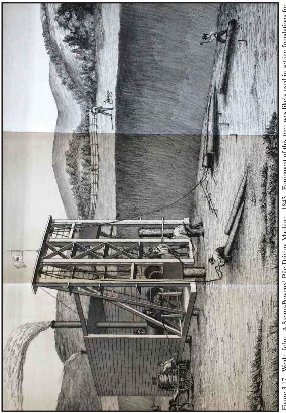
Figure 3.17. Weale, John. A Steam-Powered Pile Driving Machine. 1843. Equipment of this type was likely used in setting foundations for structures like turntables which required especially sound footings.
