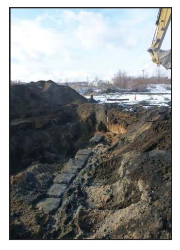
Photograph 4.2. View looking southwest showing Remedial Area 16 (PHE Area 3) with excavation in progress and the first line of stone sleepers in the process of being exposed; scales in feet (Photographer: Joshua Butchko, January 2017) [HRI Neg. #16008/D7:554].
