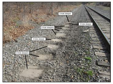
View along part of the original Camden and Amboy Railroad route showing a line of in-situ stone sleepers. Part of the original rail bed has been swept clean to show the typical configuration of the two-hole and four-hole blocks. [Source: Hunter Research, Inc.]
