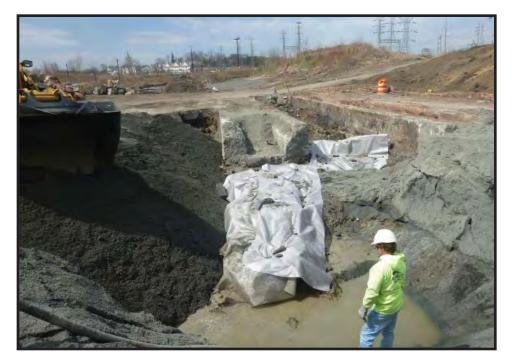
Photograph 3.41. View looking west showing the remaining portions of the mid-19th-century turntable being covered with geotextile fabric and reburied beneath gravel remedial fill (Photographer: Joshua Butchko, April 2017) [HRI Neg. #17023/D1:527].
