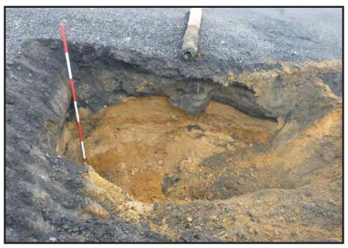
Photograph 5.1. View looking north showing Remedial Area 1 (PHE S-9) at the conclusion of excavation; no cultural features were observed; the soil profile shows a gravel surface over a thin layer of historic fill over undisturbed natural sands; scale in feet (Photographer: Joshua Butchko, January 2017) [HRI Neg. #16008/D7:380].
