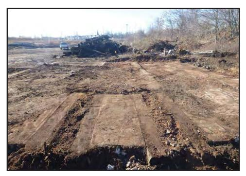
Photograph 3.13. View looking southwest across the northwestern corner of Remedial Area 15 (PHE Area 2) at an early stage of excavation; the linear features are the tops of the concrete ash pits [1, 9, 10, 12] inside the engine house [Structure 58] (Photographer: Joshua Butchko, December 2016) [HRI Neg. #16008/D6:158].
