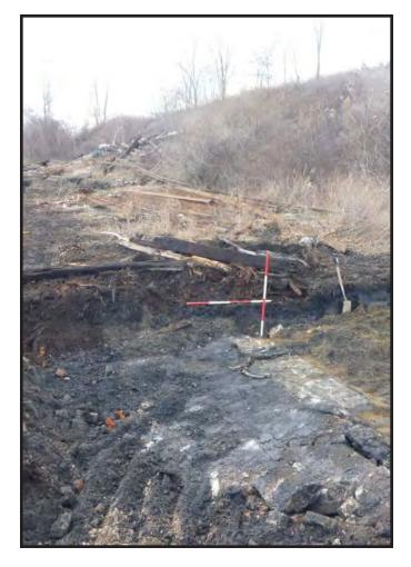
Photograph 5.20. View looking west-northwest showing the western end of Remedial Area 17 (PHE Area 1); the concrete floor and brick and stone foundation of the machine shop [Structure 43] are visible in the foreground; remediation in this area occurred within historic fill and contaminated natural sands to a depth of three feet; scales in feet (Photographer: Joshua Butchko, December 2016) [HRI Neg. #16008/D7:413].
