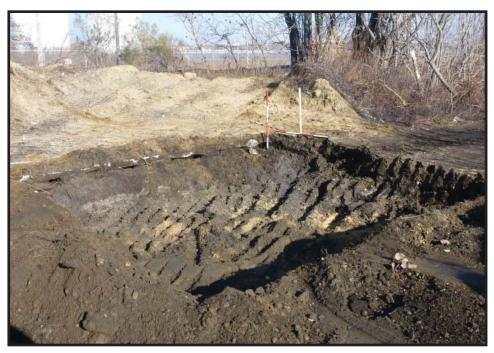
Photograph 5.5. View looking northeast showing Remedial Area 5 (PHE Area 5) at the conclusion of excavation; the concrete slab floor in the soil profile may be associated with a *circa* 1950 pump house; the soil profile shows the concrete slab over historic fill over undisturbed natural sands; remediation occurred to a depth of approximately three feet; scales in feet (Photographer: Joshua Butchko, December 2016) [HRI Neg. #16008/D5:128].
