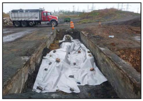
Photograph 3.46. View looking west showing the western extension of Remedial Area 15 (PHE Area 2) being prepared for backfilling; the mortared brick and stone foundations supporting the approach track leading into the mid-19th-century turntable were covered with geotextile fabric (Photographer: Joshua Butchko, April 2017) [HRI Neg. #17023/D1:702].
