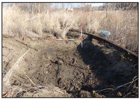
Photograph 5.7. View looking east showing Remedial Area 7 (AOC7-PHE 16) at the conclusion of excavation; no cultural features were observed within the trench; the soil profile shows gravel fill and assorted lumber; the rail track at right has been pulled aside to allow for excavation; remediation occurred to a depth of approximately two feet; scales in feet (Photographer: Joshua Butchko, December 2016) [HRI Neg. #16008/D5:167].
