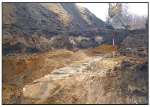
Photograph 4.3. View looking southwest showing the first line of stone sleepers set into thick layer of sand fill at the southwestern end of Remedial Area 16 (PHE Area 3); scales in feet and tenths of feet (Photographer: Joshua Butchko, January 2017) [HRI Neg. #16008/D8:070].
