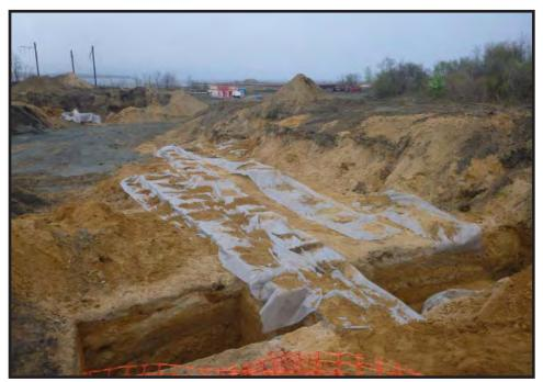
Photograph 4.16. View looking east showing the stone sleepers, masonry and gravel features in Remedial Area 16 (PHE Area 3) being buried under protective geotextile fabric before backfilling (Photographer: Joshua Butchko, April 2017) [HRI Neg. #17023/D1:824].
