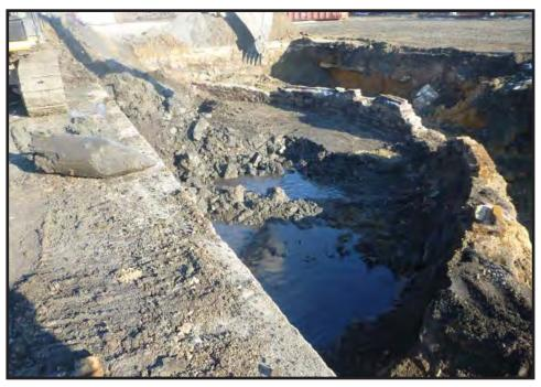
Photograph 3.24. View looking east-southeast showing the remains of the mid-19th-century turntable beneath the engine house [Structure 58] in Remedial Area 15 (PHE Area 2) following removal of its mortared brick floor and the southeasternmost wall [1] of the concrete ash pit in the center bay; a sample of one of the timber pilings from beneath the turntable floor sits on the concrete foundation at left (Photographer: Joshua Butchko, January 2017) [HRI Neg. #16008/D8:356].
