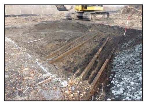
Photograph 5.2. View looking northeast showing Remedial Area 2 (PHE S-5) at the conclusion of excavation; note the two sets of rails, 4.5 feet apart, are near a switching point; remediation occurred entirely in historic fill to a depth of approximately two feet; scale in feet (Photographer: Joshua Butchko, December 2016) [HRI Neg. #16008/D5:069].
