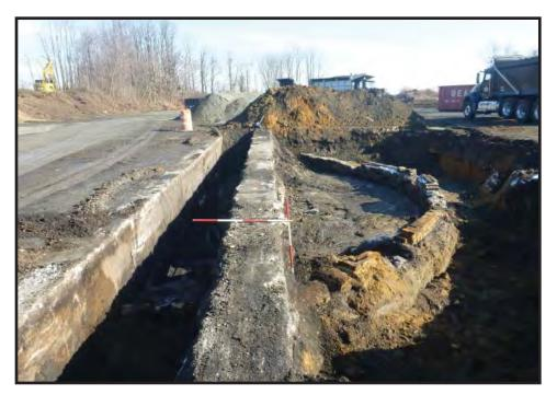
Photograph 3.23. View looking east-northeast showing the southern portion of the foundations [3, 4, 6, 16] of the mid-19th-century turntable beneath the engine house [Structure 58] in Remedial Area 15 (PHE Area 2); the concrete walls [1, 9] at center left are part of the ash pit in the central bay of the engine house overlying the turntable; scales in feet (Photographer: Joshua Butchko, January 2017) [HRI Neg. #16008/D8:290].
