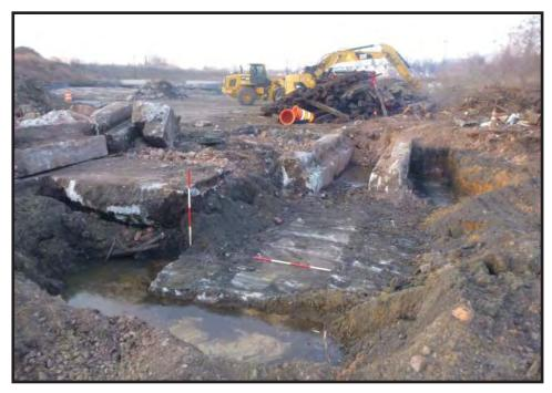
Photograph 3.18. View looking southwest showing the removal of the concrete floor [29] and ash pit [1, 2, 9] inside the northeastern end of the engine house [Structure 58] in Remedial Area 15 (PHE Area 2); scales in feet (Photographer: Joshua Butchko, December 2016) [HRI Neg. #16008/ D6:185].
