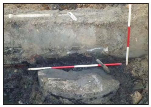
Photograph 3.10. Detailed view looking south showing the concrete pivot footing at the center of the late 19th/early 20th-century turntable [Structure 71] directly beneath the concrete drain; scales in feet and tenths of feet (Photographer: Joshua Butchko, December 2016) [HRI Neg. #16008/ D6:120].
