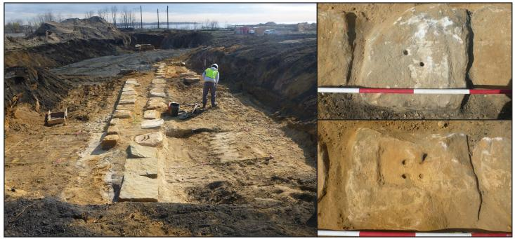
*Left:* Two lines of stone sleepers re-used from their original Camden and Amboy Railroad railbed of the early 1830s. *Right:* Close-up views of typical two-hole and four-hole stone sleepers with rectangular imprint of chair or plate. [Source: Hunter Research, Inc.]
