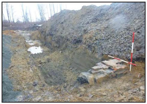
Photograph 5.17. View looking southeast showing the eastern end of Remedial Area 15 (PHE Area 2); the mortared brick and stone foundation in the foreground may be part of a carpenter's shop [Structure 90]; remediation in this area occurred within historic fill and underlying contaminated natural sands to a depth of up to six feet; scales in feet (Photographer: Joshua Butchko, December 2016) [HRI Neg. #16008/D7:347].
