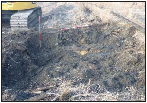
Photograph 5.11. View looking west showing Remedial Area 10 (AOC7-PHE 17) at the conclusion of excavation; no cultural features were observed; the soil profile shows historic fill over undisturbed natural sands; remediation occurred to a depth of two feet; scales in feet (Photographer: Joshua Butchko, December 2016) [HRI Neg. #16008/D5:199].
