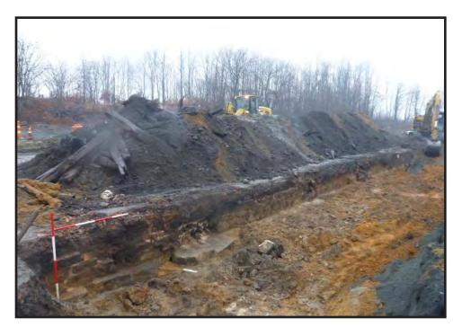
Photograph 3.15. View looking northeast showing the exterior of the stone, brick and concrete southeast foundation [39] of the engine house [Structure 58] in Remedial Area 15 (PHE Area 2); note the stone pilaster bases spaced at regular 17-foot intervals along the face of the wall; scales in feet and tenths of feet (Photographer: Joshua Butchko, January 2017) [HRI Neg. #16008/D7:309].
