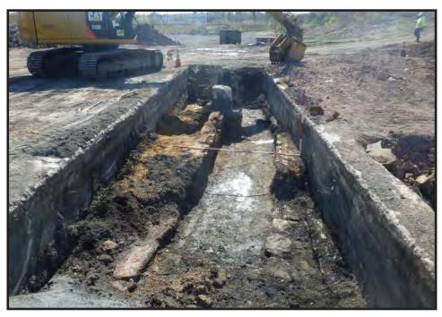
Photograph 3.42. View looking west showing the western extension of Remedial Area 15 (PHE Area 2); the two parallel mortared stone and brick foundations [20, 22] supported the approach track leading into the mid-19th-century turntable (Photographer: Joshua Butchko, April 2017) [HRI Neg. #17023/D1:593].
