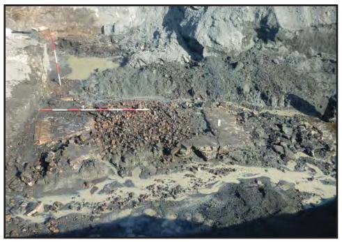
Photograph 3.32. Detailed view looking north showing the mortared brick floor [16] and rubble sub-base [6] in the inner portion of the turntable pit following removal of the ash pit's concrete floor, dewatering and clean-up; the brickwork [16] at left would have supported balance wheels beneath the middle portion of the turntable; the remnants of the pivot base footings [5] are at right; scales in feet and tenths of feet (Photographer: Joshua Butchko, April 2017) [HRI Neg. #17023/D1:220].
