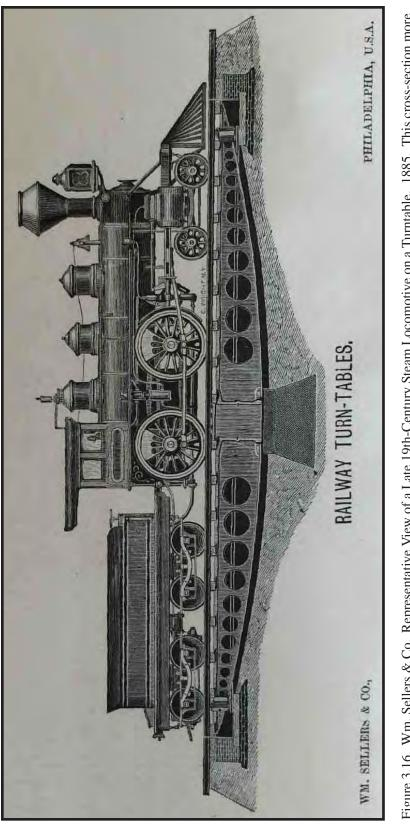
Figure 3.16. Wm. Sellers & Co. Representative View of a Late 19th-Century Steam Locomotive on a Turntable. 1885. This cross-section more likely resembles the later of the two turntables (built in 1887) documented through archaeological monitoring.
