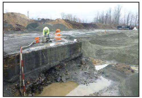
Photograph 3.25. View looking northeast showing the remains of the mid-19th-century turntable beneath the engine house [Structure 58] in Remedial Area 15 (PHE Area 2) midway through remediation; the southern portion of the turntable has been removed and replaced by gravel remedial fill; the central pivot area of the turntable still lies unexamined beneath the concrete ash pit wall [1]; scale in feet (Photographer: Joshua Butchko, January 2017) [HRI Neg. #16008/D9:018].
