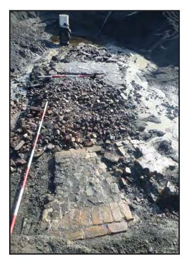
Photograph 3.33. Detailed view looking east showing the mortared brick floor [16] and rubble sub-base [6] in the inner portion of the turntable pit following removal of the ash pit's concrete floor, dewatering and clean-up; the brickwork [16] in the foreground would have supported balance wheels beneath the middle portion of the turntable; the remnants of the pivot footings [5] are beyond; scales in feet and tenths of feet (Photographer: Joshua Butchko, April 2017) [HRI Neg. #17023/D1:226].
