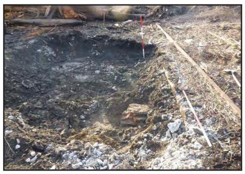
Photograph 5.9. View looking west showing Remedial Area 9 (PHE S-15) at the conclusion of excavation; the brick pier documented within the trench may relate to the structural framing of the mid-19th-century engine house [Structure 58]; the rail track and concrete slab floor would have been inside the engine house; remediation occurred entirely within historic fill to a depth of two feet; scales in feet (Photographer: Joshua Butchko, December 2016) [HRI Neg. #16008/D5:190].
