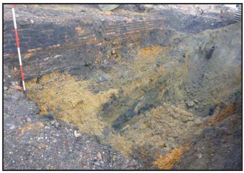
Photograph 5.13. View looking northeast showing Remedial Areas 11, 12 and 13 (AOC7-PHE 11 and AOC7-PHE 5) at the conclusion of excavation; this view shows the undisturbed contaminated natural sands beneath the boiler house/carpenter's shop [Structure 27] which were remediated to a depth of up to ten feet; scale in feet (Photographer: Joshua Butchko, January 2017) [HRI Neg. #16008/D7:394].
