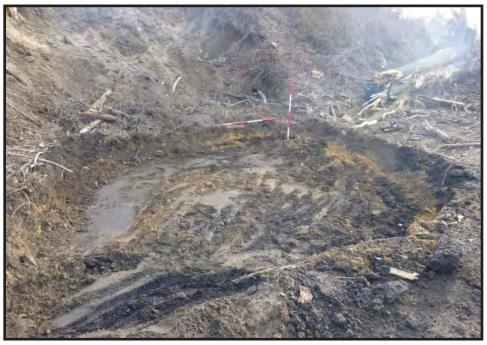
Photograph 5.3. View looking southwest showing Remedial Area 3 (PHE S-17) at the conclusion of excavation; no cultural features were observed; the soil profile shows a thin layer of fill over undisturbed natural sands; remediation occurred to a depth of approximately two feet; scales in feet (Photographer: Joshua Butchko, December 2016) [HRI Neg. #16008/D5:080].
