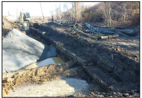
Photograph 3.7. View looking southeast showing the southwest corner of Remedial Area 15 (PHE Area 2); the linear feature along the edge of the excavation is the brick foundation supporting the northern side of the approach track leading into the late 19th/early 20th-century turntable (Photographer: Joshua Butchko, December 2016) [HRI Neg. #16008/D6:026].
