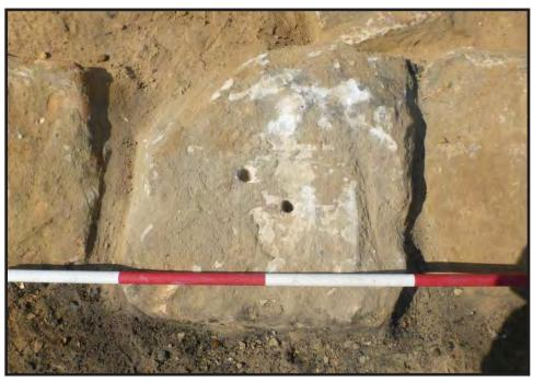
Photograph 4.7. Close-up view of typical two-hole stone sleeper showing one-inch diameter holes drilled to receive fastening trenails and spikes; traces of the rectangular outline for the setting for the locust chair or plate are just visible surrounding the drill holes; scale in feet (Photographer: Joshua Butchko, April 2017) [HRI Neg. #17023/D1:447].
