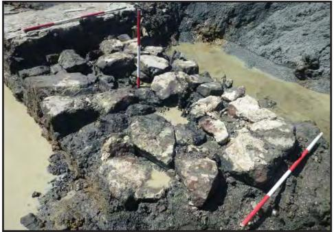
Photograph 3.31. Detailed view of the stone rubble core of the turntable's pivot footings [5] with its regularly spaced timber pilings in the center; scales in feet (Photographer: Joshua Butchko, April 2017) [HRI Neg. #17023/D1:312].
