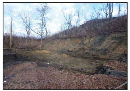
Photograph 5.25. View looking northeast showing Remedial Area 18; remediation removed one to two feet of fill and contaminated natural sands from the spit-like landform, already compromised by construction of the shooting range; scale in feet (Photographer: Joshua Butchko, December 2016) [HRI Neg. #16008/D7:277].
