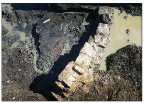
Photograph 3.34. Detailed view looking down at the outer portion of the mortared brick turntable floor [4] and perimeter wall [3] following removal of the ash pit's concrete floor, dewatering and clean-up; note the brickwork [4] in the floor that would have supported the turntable's outermost balance wheels; scale in tenths of feet (Photographer: Joshua Butchko, April 2017) [HRI Neg. #17023/D1:177].
