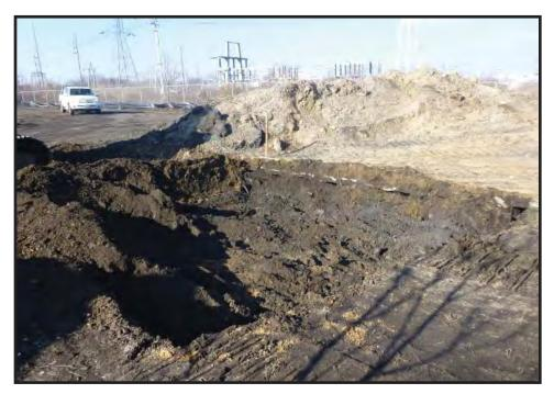
Photograph 5.4. View looking northwest showing Remedial Area 4 (PHE TP-C5) at the conclusion of excavation; a concrete slab floor close to the surface is visible in the north profile; remediation occurred entirely in historic fill to a depth of approximately four feet (Photographer: Joshua Butchko, December 2016) [HRI Neg. #16008/D5:116].
