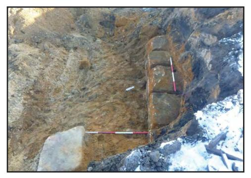
Photograph 4.4. View looking east showing the second line of stone sleepers exposed in what was then the southeastern edge of Remedial Area 16 (PHE Area 3); scales in feet and tenths of feet (Photographer: Joshua Butchko, January 2017) [HRI Neg. #16008/D8:262].
