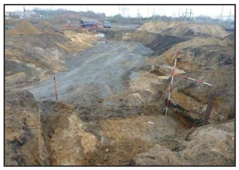
Photograph 4.11. View looking west showing the corner foundation at the northeastern end of Remedial Area 16 (PHE Area 3); the gravel remedial fill is in the center of the view with the rail bed remnants beyond; scales in feet and tenths of feet (Photographer: Joshua Butchko, April 2017) [HRI Neg. #17023/D1:686].
