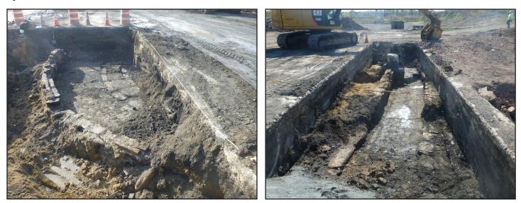
*Left:* The southern portion of the mid-19th-century turntable pit beneath the concrete floor of the engine house. *Right:* The mortared brick and stone foundation supporting the approach track leading into the mid-19th-century turntable. [Source: Hunter Research, Inc.].
