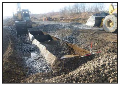
Photograph 5.18. View looking west-northwest showing a cast-iron oil tank prior to removal from the eastern end of Remedial Area 15 (PHE Area 2); scales in feet (Photographer: Joshua Butchko, December 2016) [HRI Neg. #16008/D7:151].
