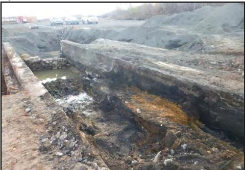
Photograph 3.39. View looking east-southeast showing early stages of excavation within and beneath the ash pit [1, 2, 9] in the western extension of Remedial Area 15 (PHE Area 2); the exterior face of the stone foundations for the brick perimeter wall [3] of the mid-19th-century turntable is visible between the concrete walls of the ash pit at the end of the excavation (Photographer: Joshua Butchko, April 2017) [HRI Neg. #17023/D1:409].
