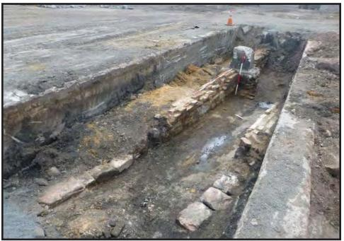
Photograph 3.45. View looking west southwest showing the western extension of Remedial Area 15 (PHE Area 2); the mortared brick and stone foundations [20, 22] supporting the approach track leading into the mid-19th-century turntable are shown at their point of maximum exposure immediately prior to backfilling with gravel remedial fill; scales in feet and tenths of feet (Photographer: Joshua Butchko, April 2017) [HRI Neg. #17023/D1:674].
