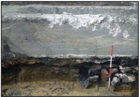
Photograph 3.35. Detailed view of part of a cross-section through the turntable base looking northnorthwest; this view shows the brick and stone foundation for the turntable perimeter wall [3] set into the underlying sandy clay and sand construction deposit [7, 15] and sealed beneath the concrete floor of the ash pit [2]; scale in feet (Photographer: Joshua Butchko, April 2017) [HRI Neg. #17023/ D1:371].
