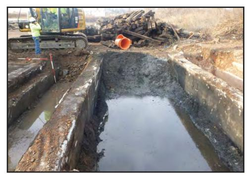
Photograph 3.19. View looking west-southwest showing the concrete ash pits inside the northeastern end of the engine house [Structure 58] in Remedial Area 15 (PHE Area 2); the ash pit in the northwestern bay [10-12] is at left, the one in the central bay [1, 2, 9] is at right; scales in feet (Photographer: Joshua Butchko, December 2016) [HRI Neg. #16008/D6:207].
