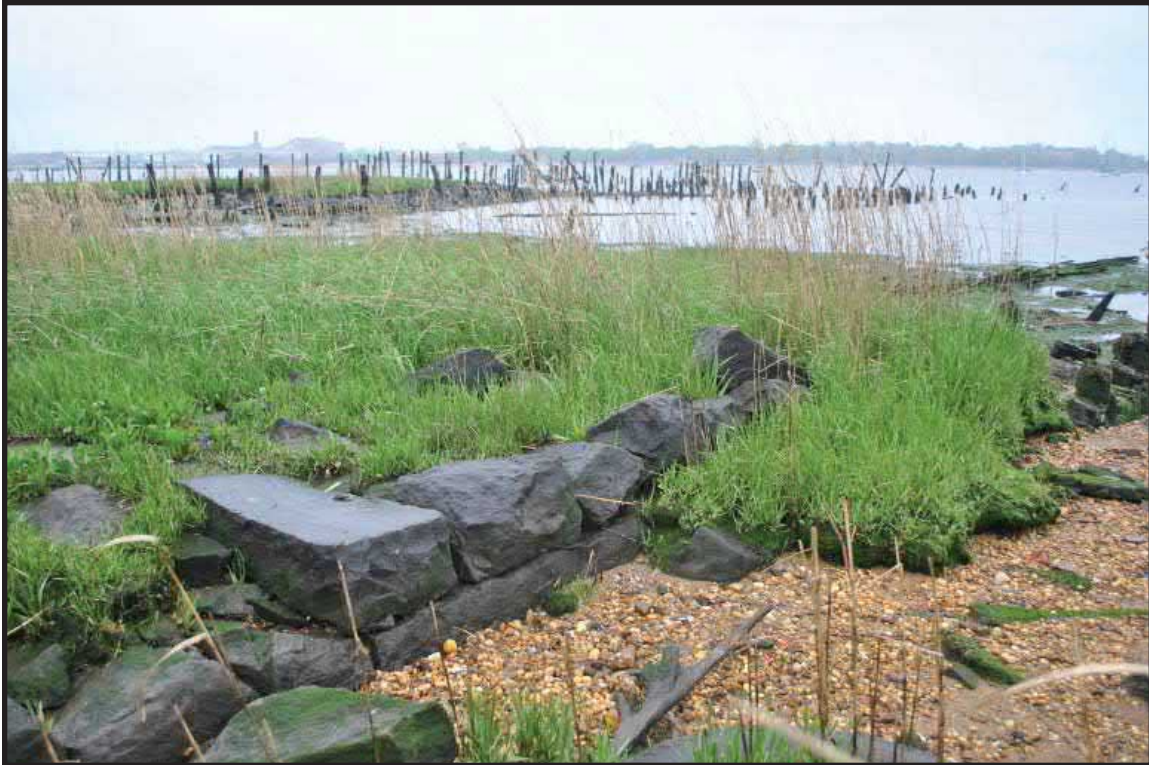
Photograph 7.7. View looking northeast showing the massive dressed stone masonry forming the onshore facing of the southeastern side of the 1870s Pennsylvania Railroad structure that supported additional sidings and a new freight house added to the existing Camden and Amboy Railroad passenger piers (Photographer: Patrick Harshbarger, May 2012) [HRI Neg. #11027/D1:19].
