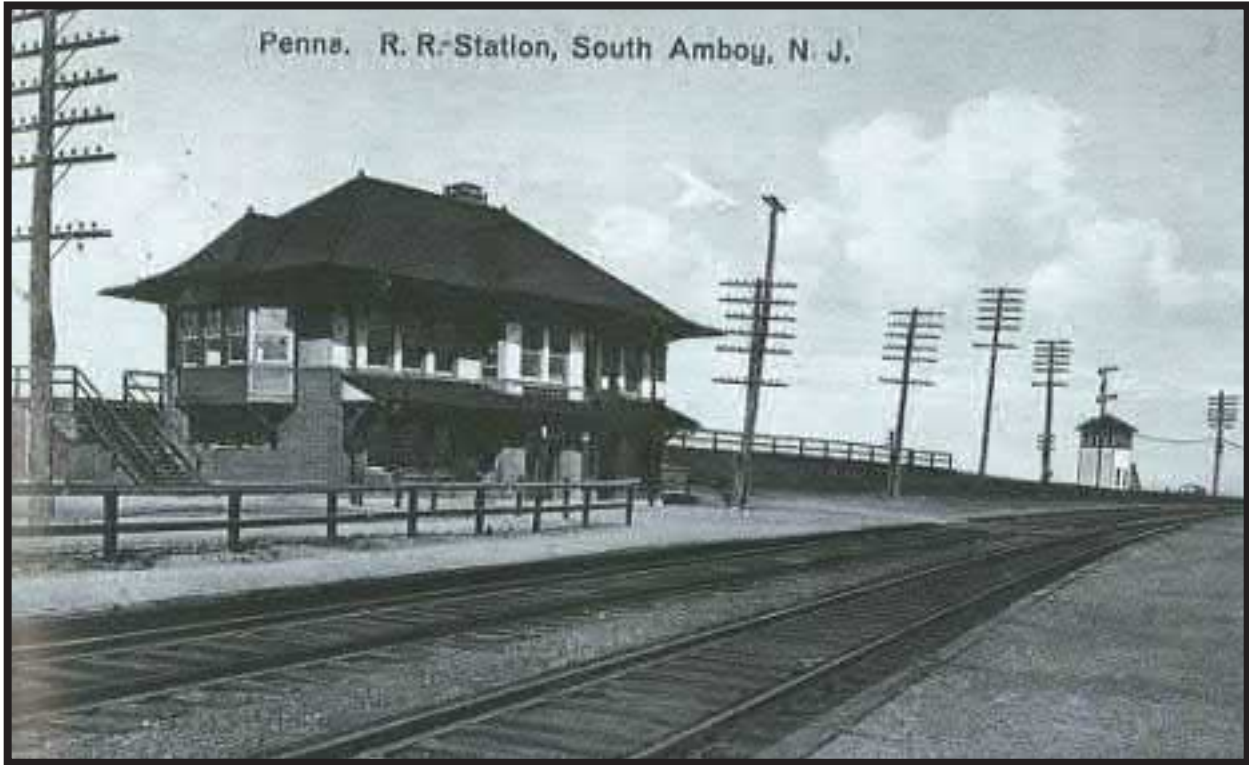
Photograph 5.15. Junction Station. South Amboy, New Jersey. Circa 1910 (Source: Francy 1998).
