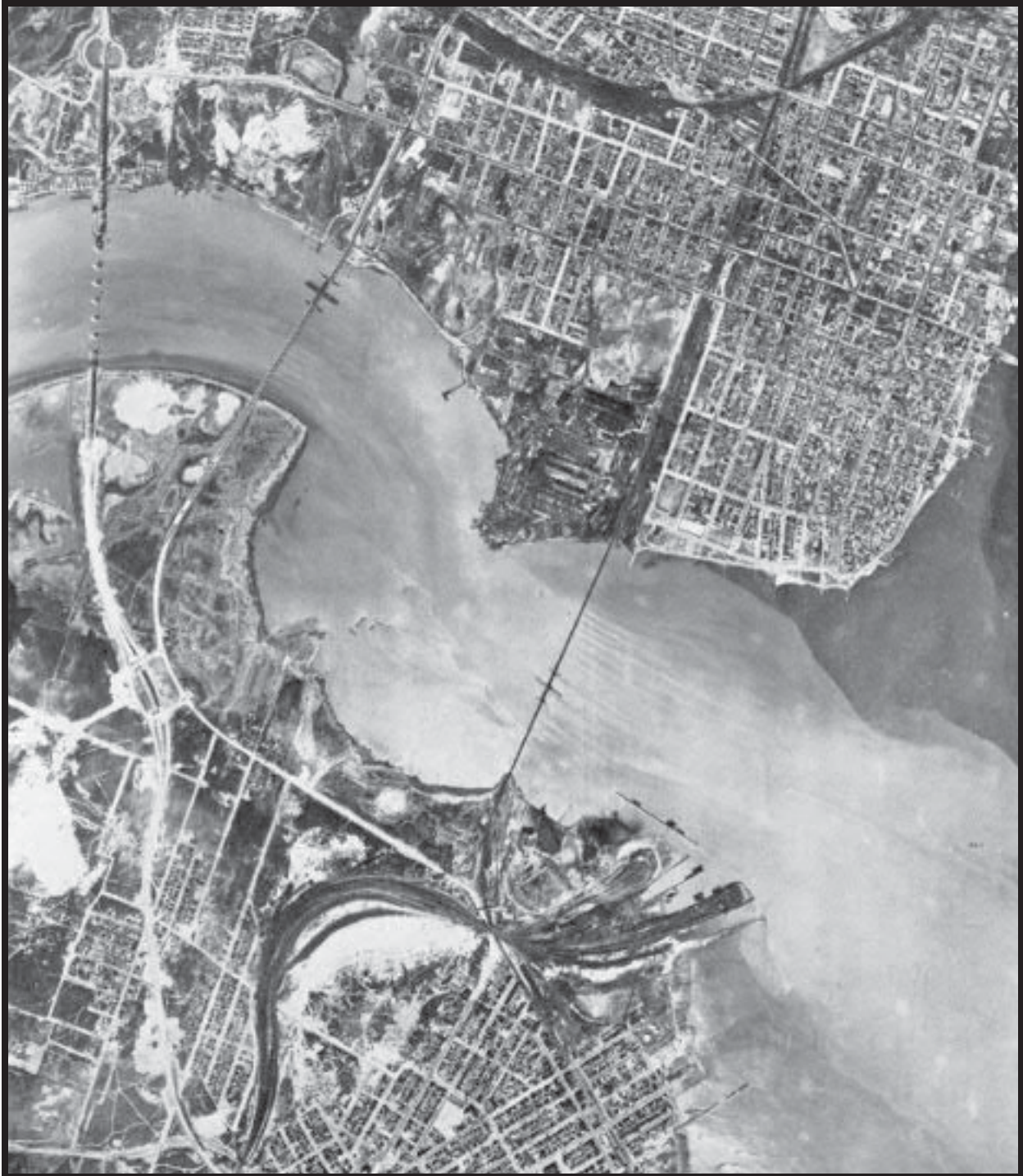
Photograph 5.27. Aerial view of the mouth of the Raritan River. Circa 1941 (Source: Journal of Industry and Finance , April 1941).
