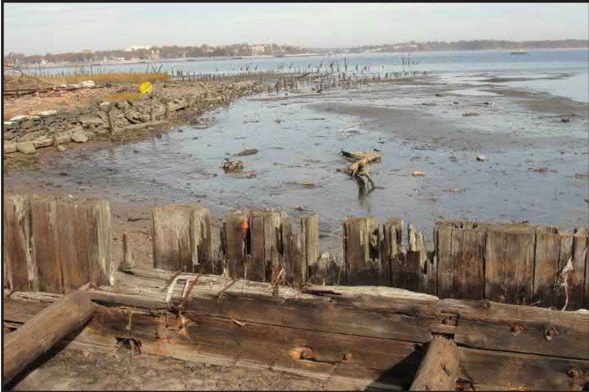
Photograph 7.11. General view looking east showing the site of the 19th-century Camden and Amboy Railroad and Pennsylvania Railroad piers and terminals. The timbering in the foreground is Pennsylvania Railroad-era bulkheading, possibly from the early 20th-century and associated with modifications related to the construction of the explosives or powder pier in 1917-18, fragmentary posts of which remain in the middle of the view (Photographer: Ian Burrow, October 2012) [HRI Neg. #11027/D5:DSC03613].
