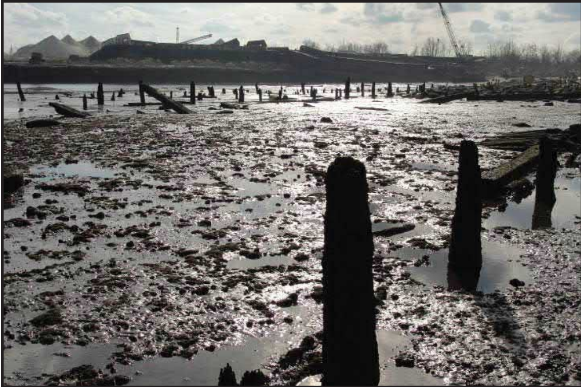
Photograph 7.9. View looking south showing the remains of the circa 1917-1950 explosives or powder pier, seen at low tide from the alignment of one of the 1870s Pennsylvania Railroad structures which supported additional sidings and the new freight house. The larger angled and vertical timbers are apparently part of the original wider explosives pier. This had been narrowed by 1950, possibly as a result of the 1923 explosion. The 1950 part of the pier is represented by the rather shorter posts beyond. Pier A (Westmoreland) is at rear, with several large barges washed onto it by Hurricane Sandy (Photographer: Ian Burrow, October 2012) [HRI Neg. #11027/D5:DSC03625].
