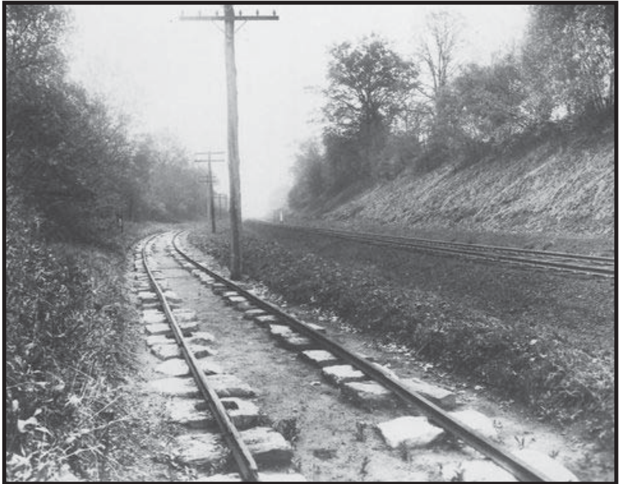
Photograph 5.6. Camden and Amboy Railroad track on stone sleepers near Jamesburg, New Jersey. Circa 1890 (Source: Smithsonian Institution Photograph Collections [Neg. # 21243-B]).
