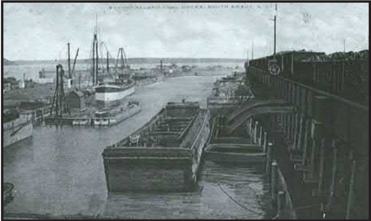
Photograph 5.17. Westmoreland coal pier, South Amboy, New Jersey. Circa 1900 (Source: Francy 1998).
