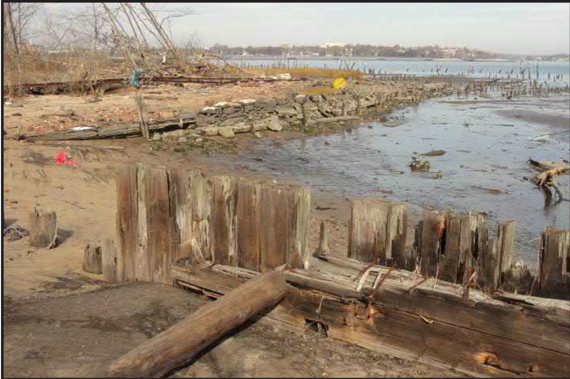
Photograph 7.12. View looking north-northeast showing the timber and stone revetment probably placed after 1950 to stabilize the shoreline after the 1950 explosion that destroyed the explosives pier. The stones include a number of Camden and Amboy Railroad-era stone sleepers which should be salvaged and used for interpretive purposes at the new ferry terminal (Photographer: Ian Burrow, October 2012) [HRI Neg. #11027/D5:DSC03614].
