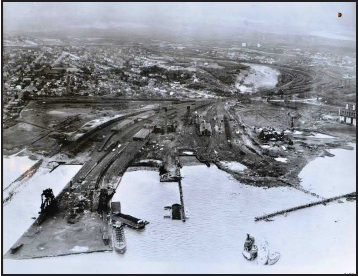
Photograph 5.33. Aerial view of the South Amboy ferry terminal, looking west, showing damage from the explosion of May 19, 1950 (Source: Pennsylvania Railroad Photographs Collection).
