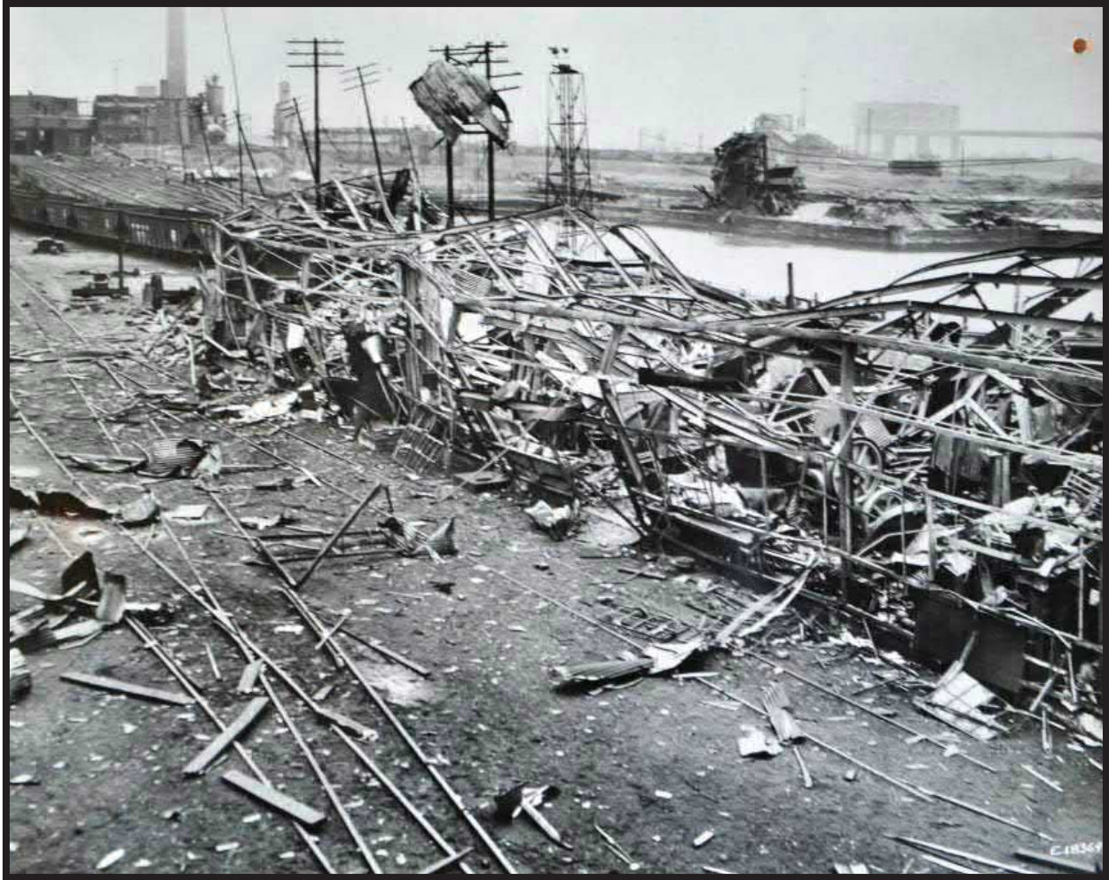
Photograph 5.35. Photograph, looking west, showing damage to the machine shop on the coal handling pier from the explosion of May 19, 1950 (Source: Pennsylvania Railroad Photographs Collection).
