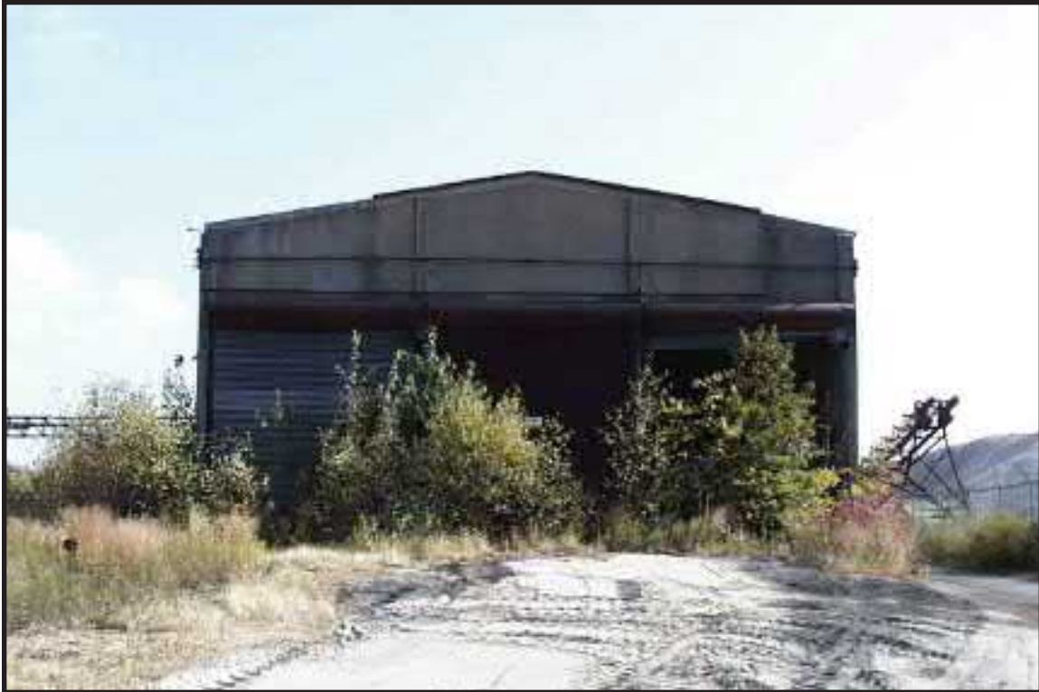
Photograph 6.4. View looking west showing the western portal of the 1916 shed (Photographer: Ian Burrow, October 2001) [HRI Neg. #01005/D3:1].
