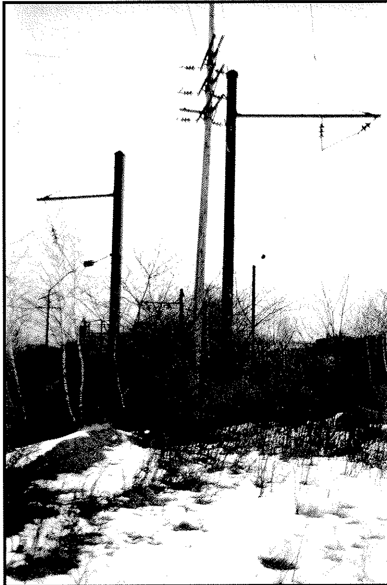
Plate 5. Bracket Arm Catenary Structures C20 and C21. View facing northeast (Photographer: Ian Burrow, December 2002). [Hunter Research Inc. Negative 02081/1:10].
