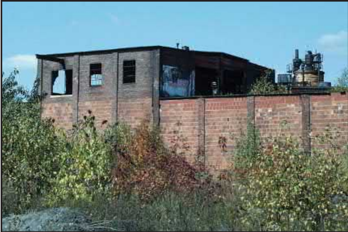
Photograph 6.3. View looking northwest showing detail of the superstructure of the 1911 shed (Photographer: Ian Burrow, October 2001) [HRI Neg. #01005/D3:14].
