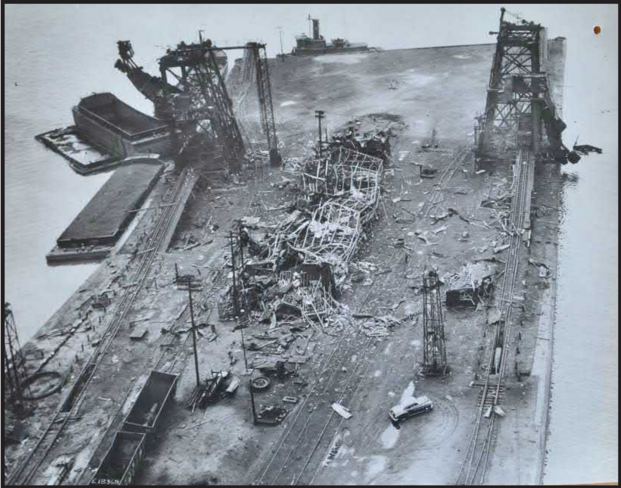
Photograph 5.34. Aerial view, looking down on the coal handling pier, showing damage from the explosion of May 19, 1950 (Source: Pennsylvania Railroad Photographs Collection).
