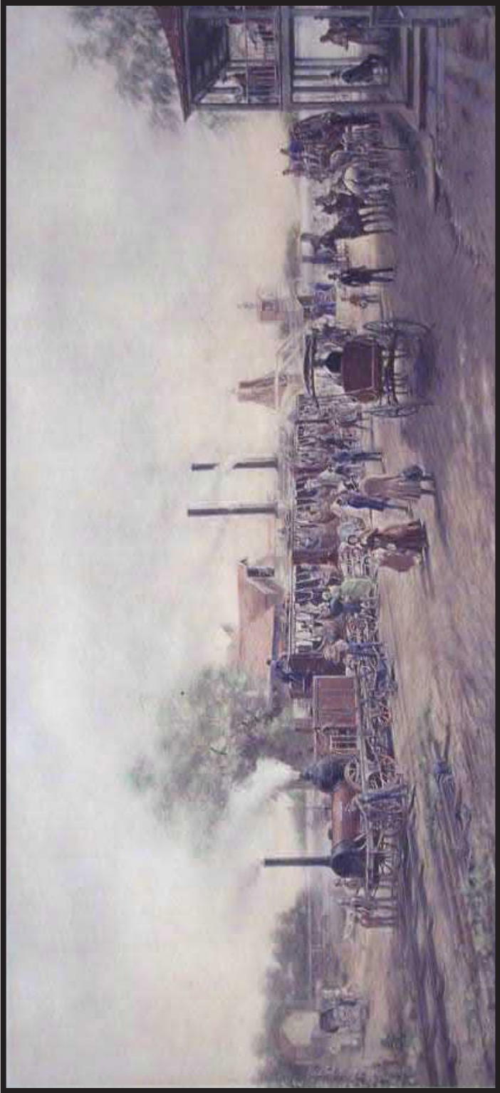
Figure 5.4. Henry, Edward Lamson. The Camden and Amboy Railroad with the Engine Planet in 1834 . 1904. Henry prided himself on accuracy of detail, capturing the bustle and excitement of passengers boarding a train at Bordentown. The cars, resembling old-fashioned stagecoaches, were the first used on the Camden and Amboy. These quickly evolved in the late 1830s to the more familiar box-shape of the American passenger car (Source: Newark Public Library).
