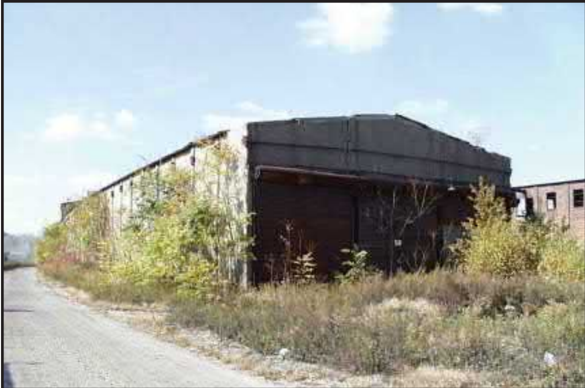
Photograph 6.5. View looking west-northwest showing the eastern end of the 1916 shed, with part of the 1911 shed visible at right (Photographer: Ian Burrow, October 2001) [HRI Neg. #01005/D3:13].
