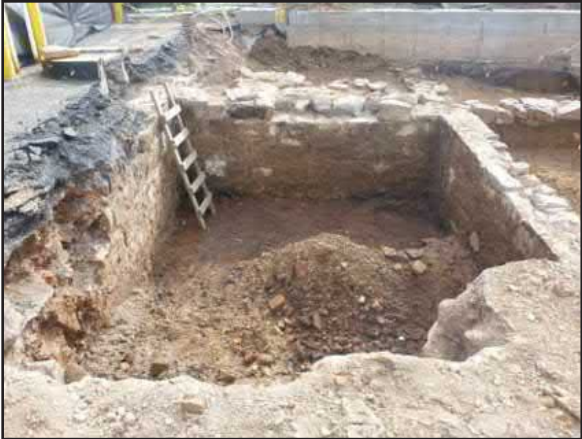
Photograph 5.8. View looking south across the basement [110-113] beneath the front portion of the northernmost dwelling at 71 Halsey Street. The sidewalk along the west side of Halsey Street is at upper left (Photographer: Joshua Butchko, March 2017) [HRI Neg.# 17002-17017/D1:493].
