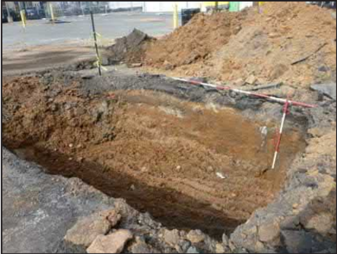
Photograph 3.9. View facing northeast showing the north wall profile of Test Pit 2. Scales in feet (Photographer: Josh Butchko, February 2017) [HRI Neg.# 17002-17017/D1:160].
