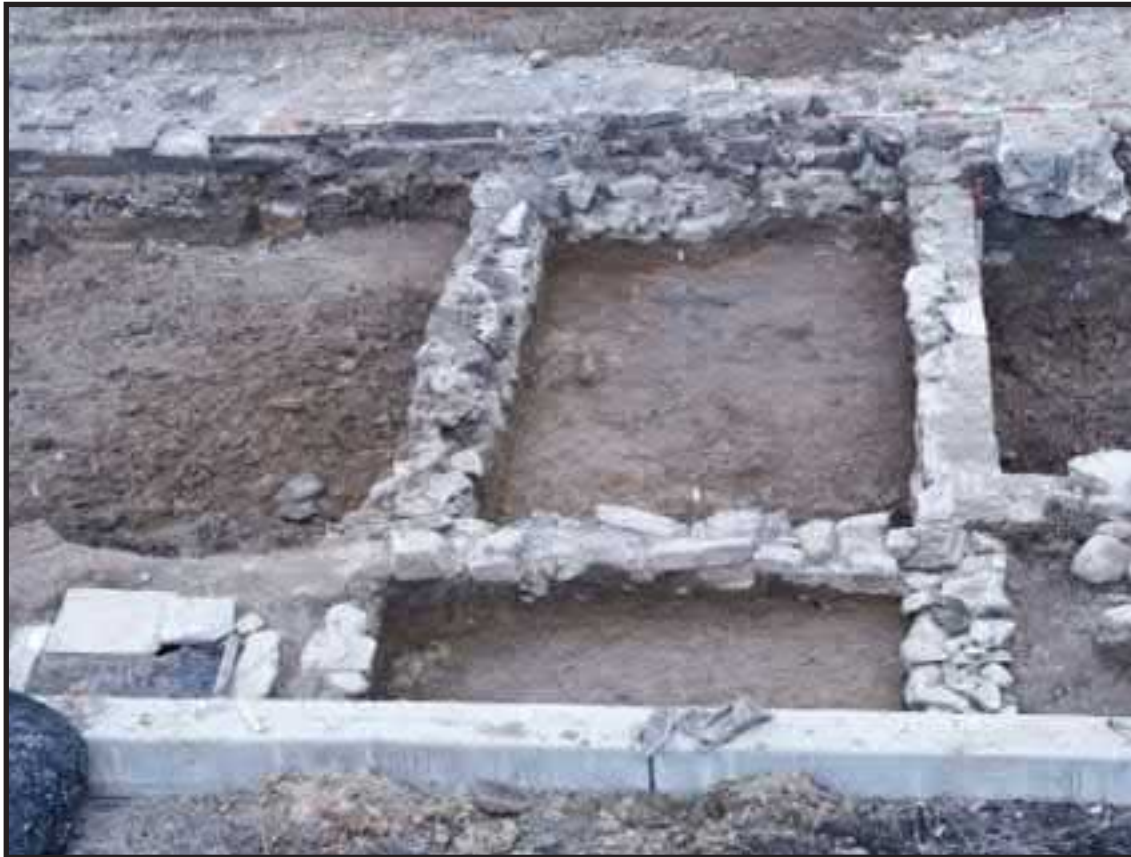
Photograph 5.9. View looking north showing the mortared stone foundations [113, 119-122] for the rear wings of the two-section dwelling at 71 Halsey Street. The rectangular space at center defines the shoe shop in the rear wing of the northernmost dwelling. At lower left is a stone-lined cistern [125, 126] positioned at the rear of the southernmost dwelling (Photographer: Joshua Butchko, March 2017) [HRI Neg.# 17002-17017/D2:178].
