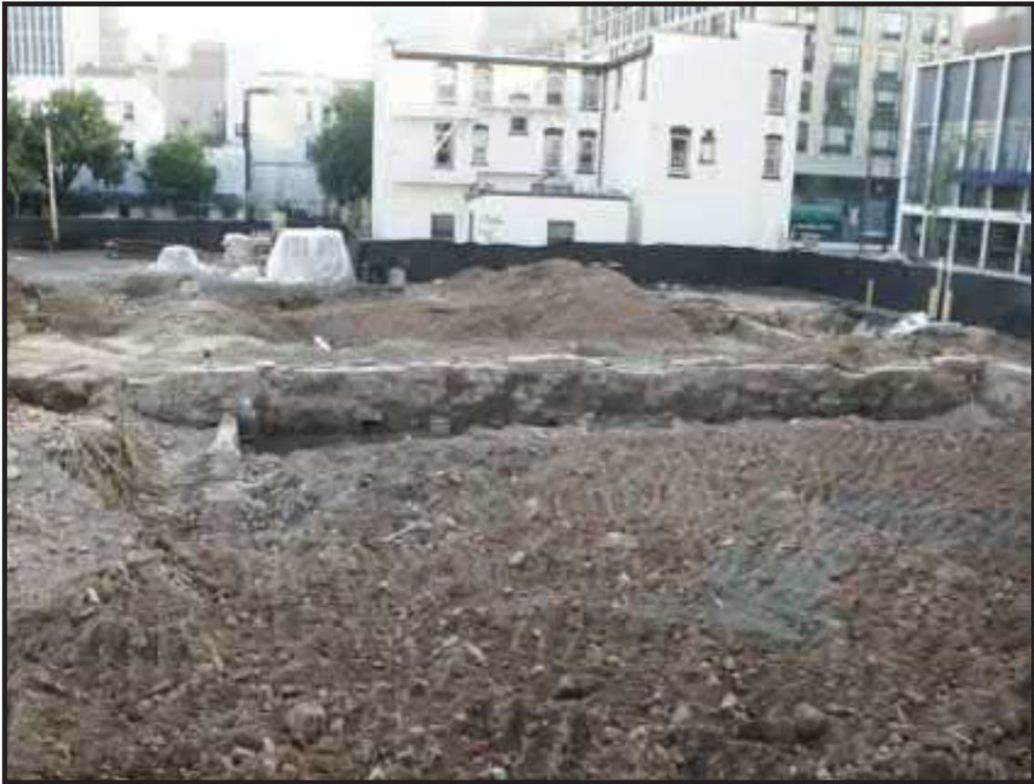
Photograph 4.4. View facing north showing the north foundation wall [1163] of the Halsey Street Methodist Episcopal Church. Note the voids set into the base of the wall and the inverted arches under the windows; scales in feet (Photographer: Michael Brown, July 2017) [HRI Neg.# 17033/D6:2055].
