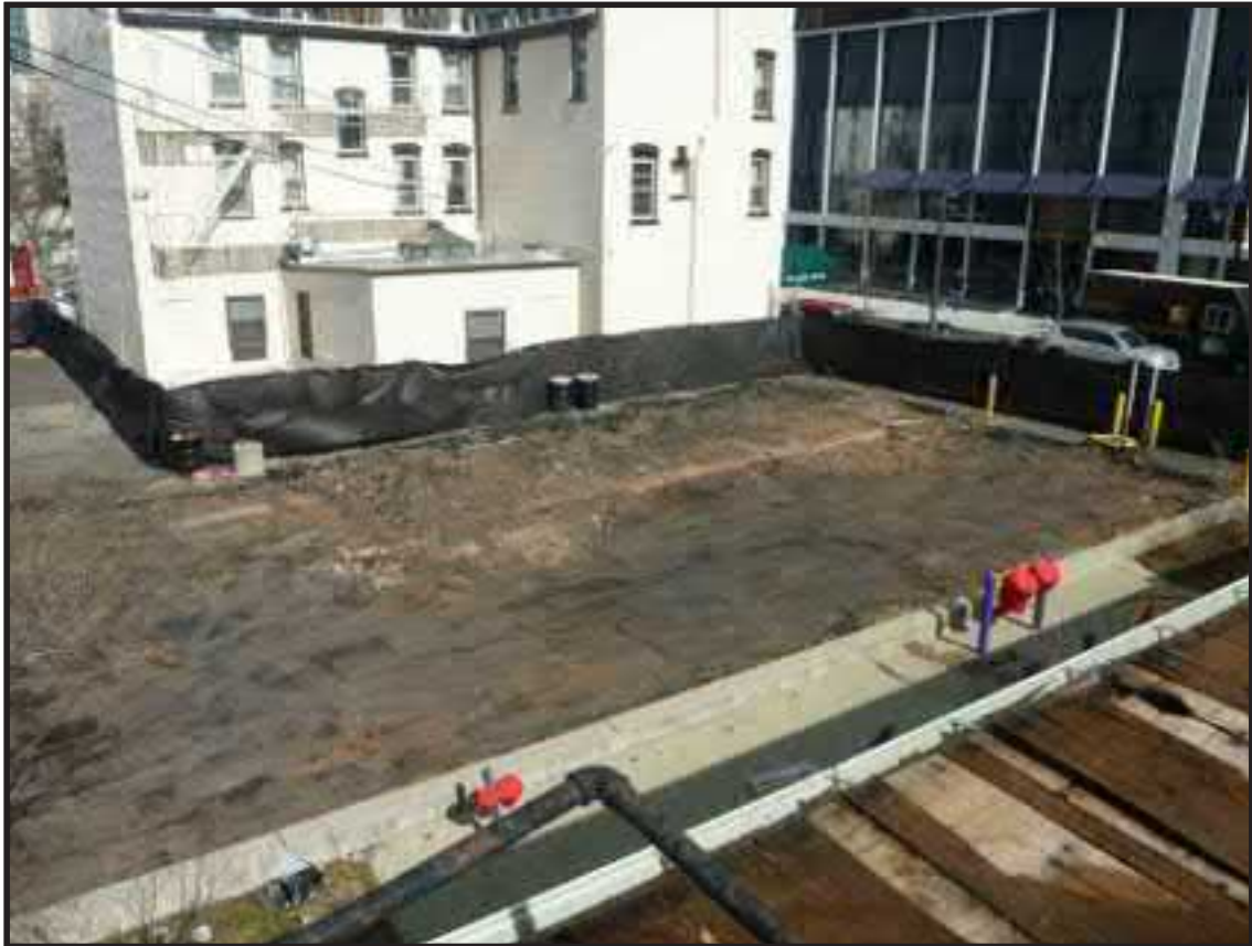
Photograph 5.1. View looking northeast showing the mortared brick foundations [103, 107] of the dwelling at 69 Halsey Street. A line of slate slabs [109] extends from the rear of the house and led to a stone-lined privy [330] (Photographer: Joshua Butchko, March 2017) [HRI Neg.# 17002-17017/D1:382].
