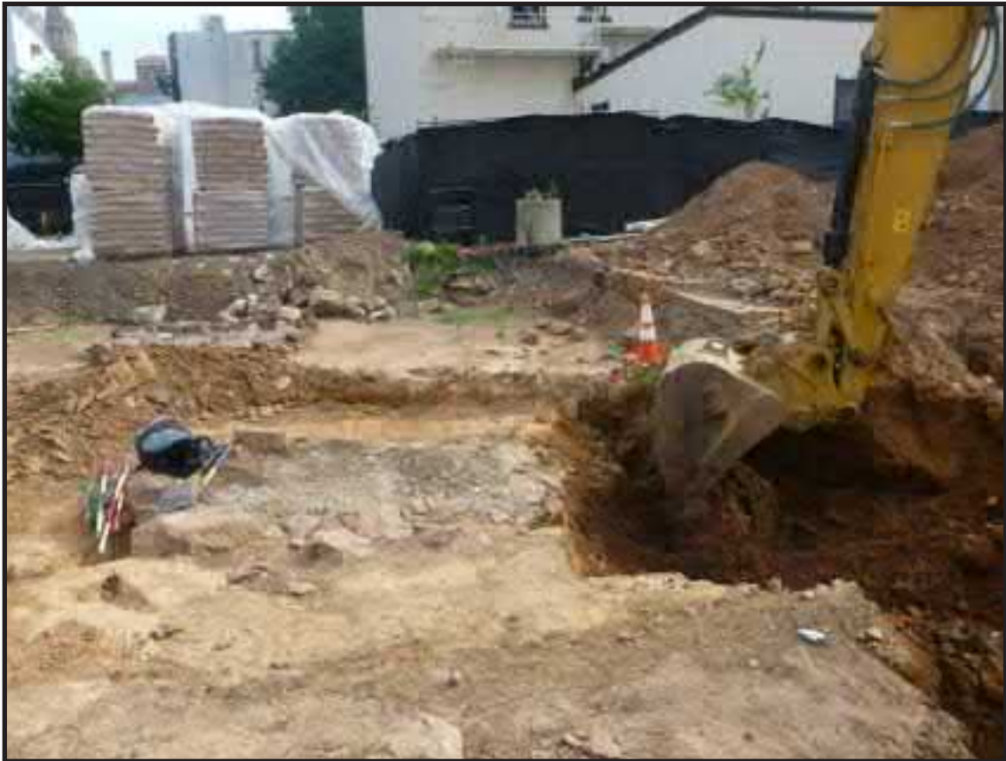
Photograph 5.11. View looking north across the stone-lined privy [1081] identified in the rear yard behind the northernmost dwelling at 71 Halsey Street. The privy to the rear of 69 Halsey Street is visible beyond and to the left, and the rear wall of the dwelling at 69 Halsey Street is beyond the backhoe bucket; scales in feet (Photographer: Joshua Butchko, July 2017) [HRI Neg.# 17033/D8:016].
