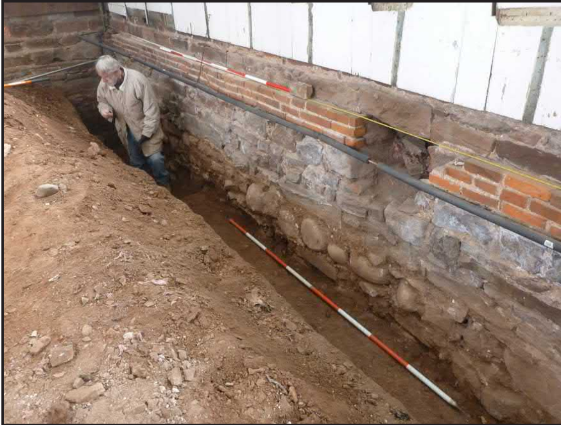
Photograph 3.14. View looking southeast showing the eastern end of Trench 2. The ghosting in the whitewashed wall covering at top shows where the ends of pews were secured to the south wall of the church. The top surface of the three courses of brick masonry represents the first-floor level of the auditorium. The rectangular recess in the foundation is a joist pocket for one of the principal members of the first-floor framing. Note that, unlike with the western section of this foundation in Trench 2, there is no offset in the masonry at the base of the foundation (cf. Photograph 3.13). Scales in feet (Photographer: Joshua Butchko, February 2015) [HRI Neg. #15001/D3:198].
