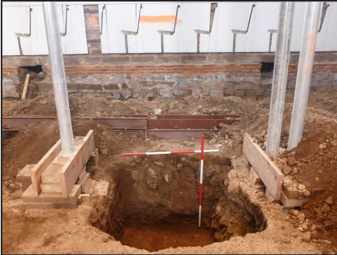
Photograph 3.22. View facing north showing the north profile of the excavation for Pier Footing 1. Behind and to the left of the vertical scale pole is the robber trench resulting from the removal of the foundation for the east wall of the original church built in 1767. Note that in this view the center wood column along the northern side aisle has been temporarily removed (and its mortared stone foundation permanently removed), pending a replacement footing being installed in the excavated pit. Scales in feet (Photographer: Joshua Butchko, February 2015) [HRI Neg. #15001/D3:157].
