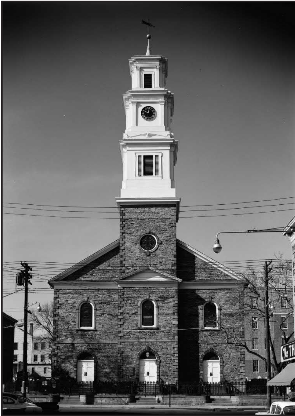
Photograph 1.1. View looking west across Neilson Street showing the east (front) façade of the First Reformed Church of New Brunswick. 1960. Source: HABS 1960.
