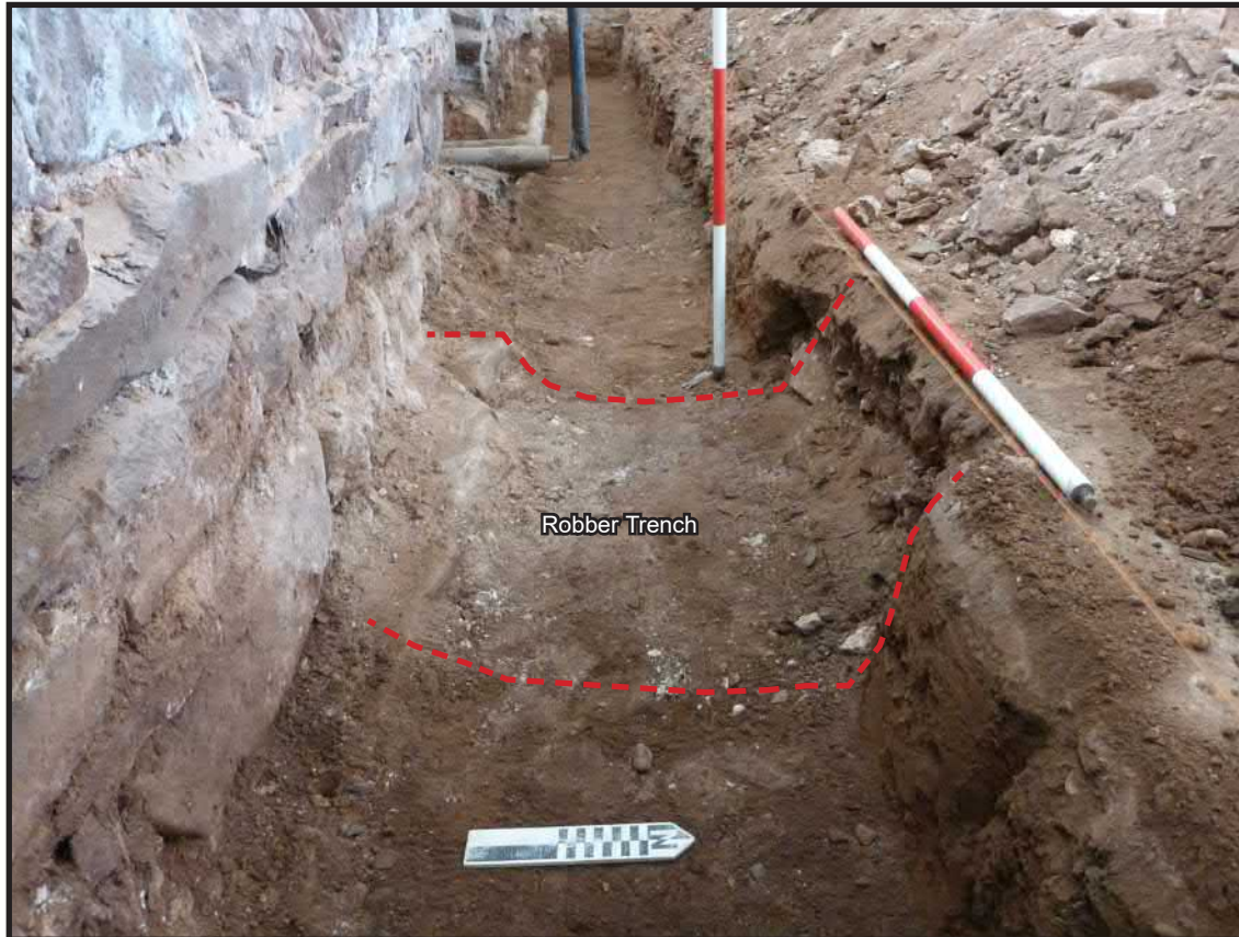
Photograph 3.12. View looking west showing the central portion of Trench 2 fully excavated. At left is the stone masonry of the church's south wall foundation. In the north wall (at right below the horizontal scale pole) and floor of the trench is a concentration of mortar, plaster and rubble thought to be the fill of the robber trench reflecting the removal of the foundation for the east wall of the original church of 1767. The lower part of the foundation extending west from the robber trench (i.e., away from the viewer) is offset and on a slightly different alignment to the masonry above and is considered to be a re-used, in-situ segment of the north foundation of the original church of 1767. Scales in feet and tenths of feet (Photographer: Joshua Butchko, February 2015) [HRI Neg. #15001/D2:232].
