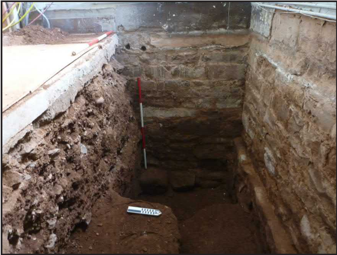
Photograph 3.32. View looking west showing the western end of the Utility Excavation Area in the church foyer. At right is the foundation for the north wall of the church with a stone offset near the base. In the center is the east face of the foundation for the interior wall separating the foyer from the auditorium. Scales in feet and tenths of feet (Photographer: Joshua Butchko, August 2015) [HRI Neg. #15004/D2:040].
