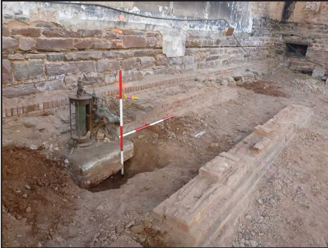
Photograph 3.4. View looking northwest showing the partially removed foundations for the dais in the sanctuary. The main west wall of the church is in the background with a brick capping on the foundation offset. The top of the brick capping is considered to represent the original first-floor level of the dais, which was later raised to a higher level, probably to allow for installation of a new pipe organ powered by a water engine. A brick foundation has also been built up against the offset of the church's west wall foundation with the water engine for the pipe organ set on a bluestone slab inserted roughly midway along its course. A second mortared brick on stone foundation in the foreground provides additional support for the dais and organ. Scales in feet and tenths of feet (Photographer: Joshua Butchko, January 2015) [HRI Neg. #15001/D1:161].
