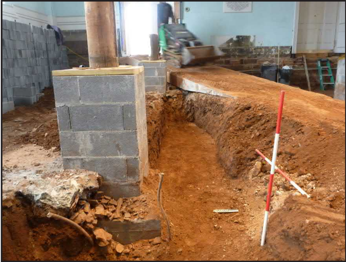
Photograph 3.19. View looking east showing the south profile of Trench 6 at right and the concentration of mortar and stone rubble interpreted as a robber trench reflecting the removal of the foundation for the east wall of the original church built in 1767. Pier Footing 1 has been recently installed at left, replacing the mortared stone foundation that had originally supported the wooden column above. Scales in feet and tenths of feet (Photographer: Joshua Butchko, March 2015) [HRI Neg. #15001/D8:142].
