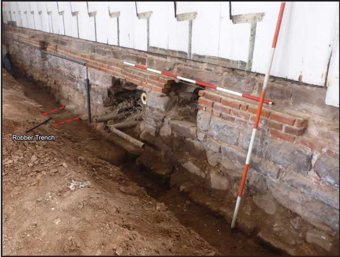
Photograph 3.13. View looking southeast showing the western end of Trench 2. The ghosting in the whitewashed wall covering at top shows where the ends of pews were secured to the south wall of the church. The top surface of the three courses of brick masonry represents the first-floor level of the auditorium. The two higher rectangular recesses in the foundation are joist pockets for two of the principal members of the first-floor framing. The larger void with the protruding pipes is the result of a later intrusion caused by the installation of utilities. At the base of the vertical scale pole is an offset in the foundation which is on a slightly different alignment to the masonry above. This offset is considered to be a re-used, in-situ segment of the south foundation of the original church of 1767. The offset was absent to the east beyond the robber trench reflecting the removal of the foundation for the east wall of the original church of 1767. Scales in feet and tenths of feet (Photographer: Joshua Butchko, February 2015) [HRI Neg. #15001/D3:188].
