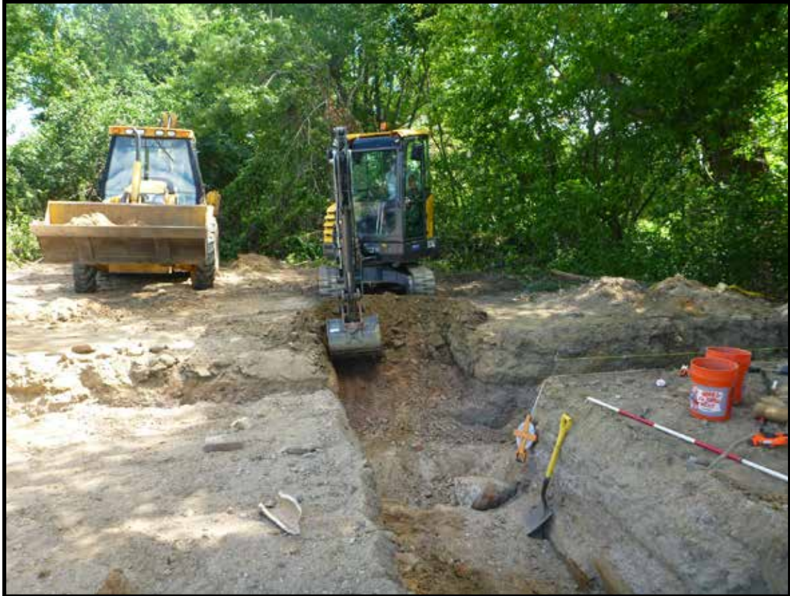
Photograph 3.7. View looking southeast during machine excavation of Trench 102 (Photographer: Joshua Butchko, August 2016) [HRI Neg. #16034/D1:045].
