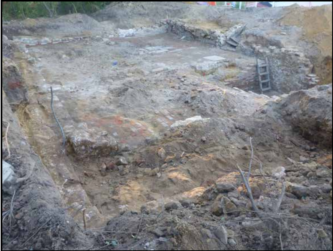
Photograph 3.14. View looking northwest showing final view of the Borton/Ballinger Farm House basement floor plan (Photographer: Joshua Butchko, September 2016) [HRI Neg. #16034/D3:363].
