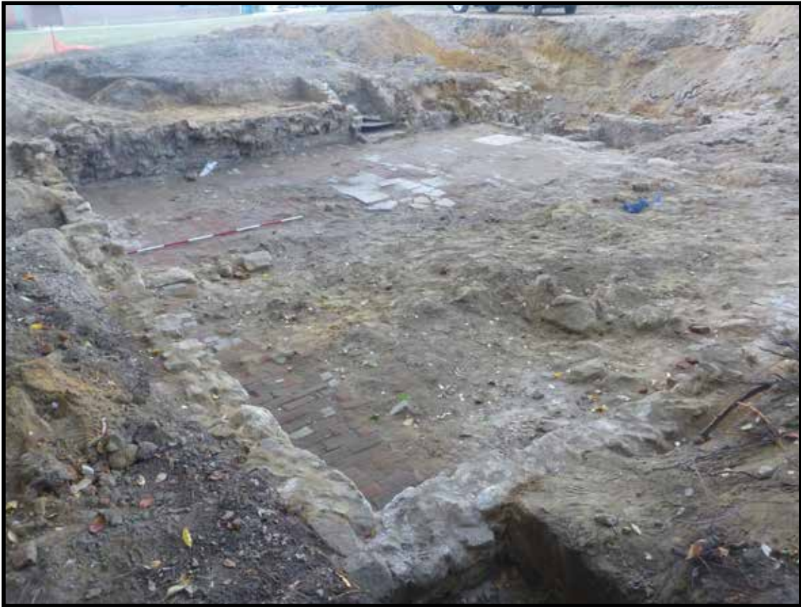
Photograph 3.15. View looking northeast showing final view of the Borton/Ballinger Farm House basement floor plan (Photographer: Joshua Butchko, September 2016) [HRI Neg. #16034/D3:384].
