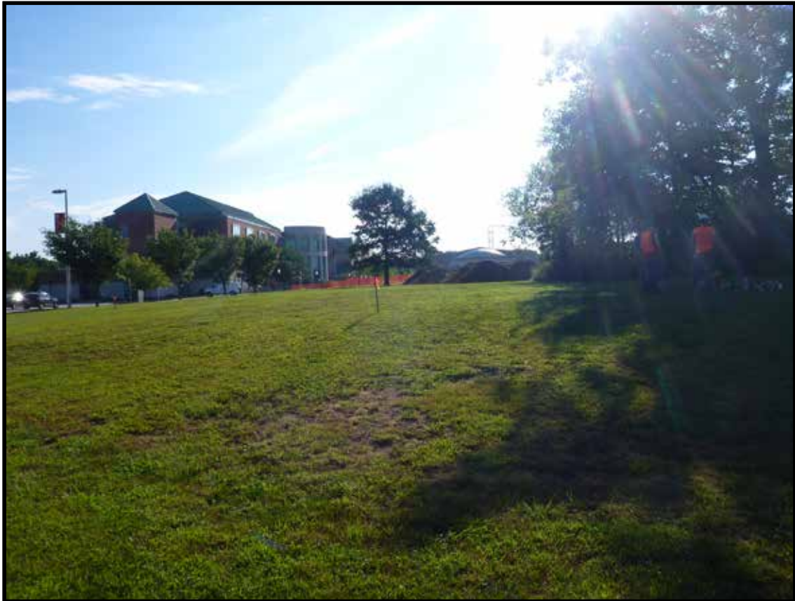
Photograph 3.1. View looking southeast of Borton/Ballinger Farmhouse Area prior to the start of excavation (Photographer: Joshua Butchko, August 2016) [HRI Neg. #16034/D1:003].
