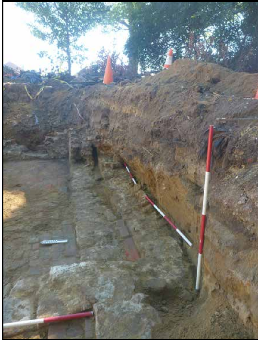
Photograph 3.23. View looking west showing foundations of possible earlier structure truncated by the original house foundation (Photographer: Joshua Butchko, September 2016) [HRI Neg. #16034/D3:310].
