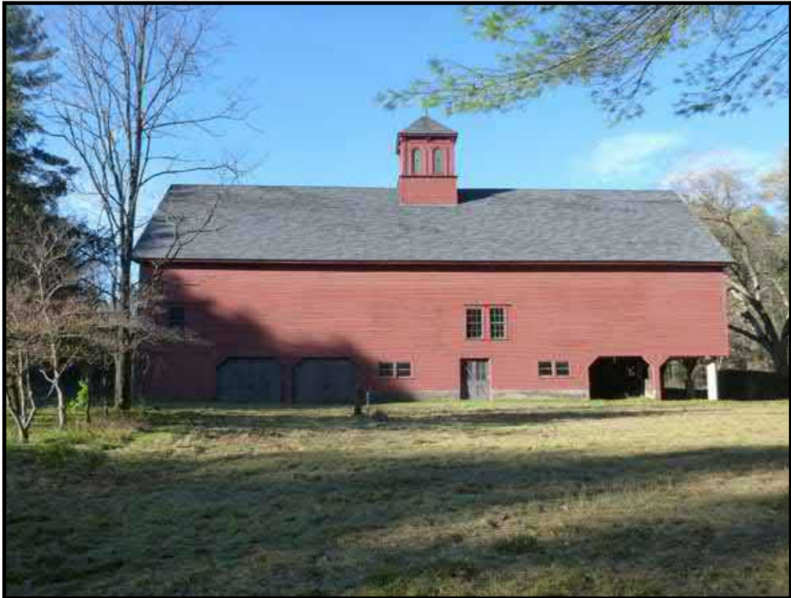
Photograph 6.20. View north showing the Barn (photographer: James Lee, November 2016) [HRI Neg.#16048/D2-95].
