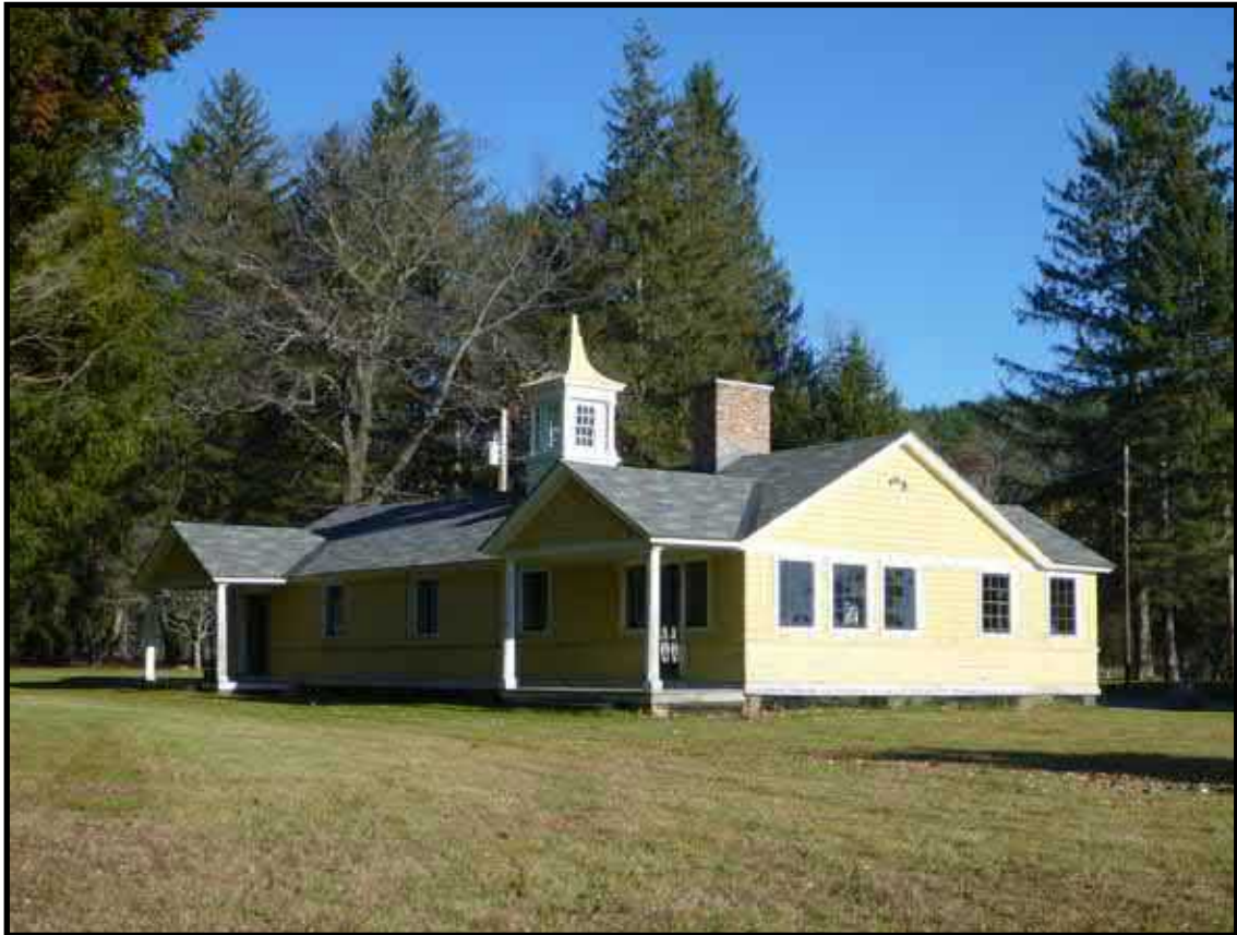
Photograph 6.11. View southeast showing the Dance Hall (photographer: James Lee, November 2016) [HRI Neg.#16048/D2-139].
