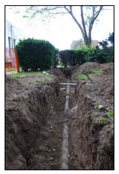
Photograph 3.40. Trench 1: view looking west showing the continuation of the trench where existing utility trenches were re-used by the contractor (Photographer: Joshua Butchko, June 2012) [HRI Neg.#11063/D20-14].
