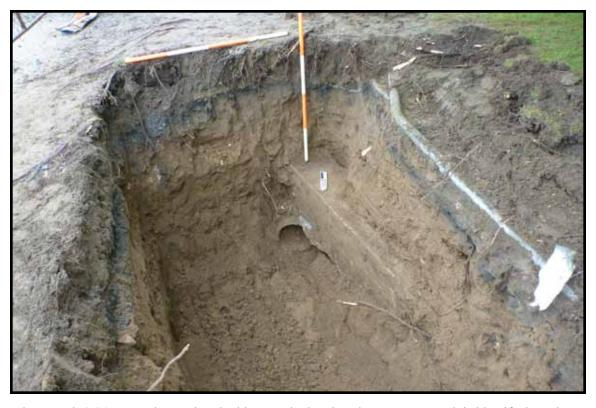
Photograph 3.34. Trench 1: view looking south showing the concrete conduit identified northeast of the flag plaza; scales in feet and tenths of feet (Photographer: Joshua Butchko, May 2012) [HRI Neg.#11063/D15-154].
