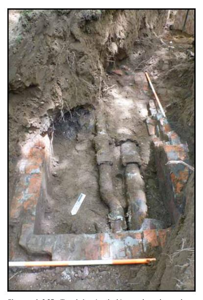
Photograph 3.27. Trench 1: view looking south southwest showing the brick utility pipe enclosure adjacent to the officer's house foundation; scales in feet and tenths of feet (Photographer: Joshua Butchko, May 2012) [HRI Neg.#11063/D15-111].
