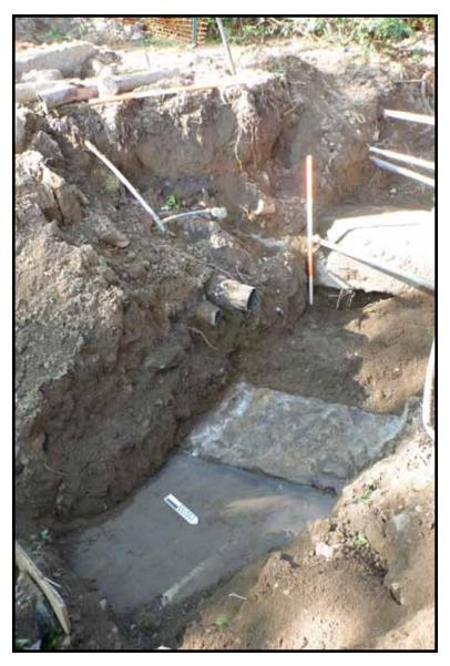
Photograph 3.32. Trench 1, Westward Extension: view looking southwest showing the southwest foundation [21] of the officer's house and a concrete-encased utility [22]; scales in feet and tenths of feet (Photographer: Joshua Butchko, May 2012) [HRI Neg.#11063/D16-40].
